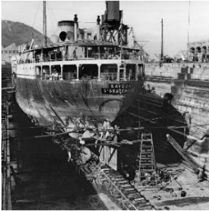
The dry dock at Taikoo Dockyard, completed in 1907, was then able to take the world's largest ships. Photo taken by Hedda Morrison ©2024: President and Fellows of Harvard College
